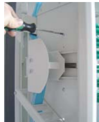
Releasing the patch cord
