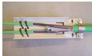
Installed tubes and cable
