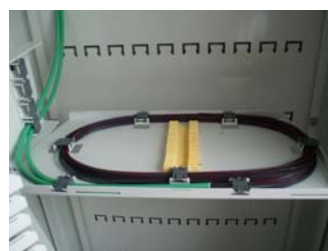
Tubes and ribbons prepared in the cassette
