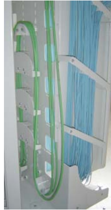
Releasing the cable
