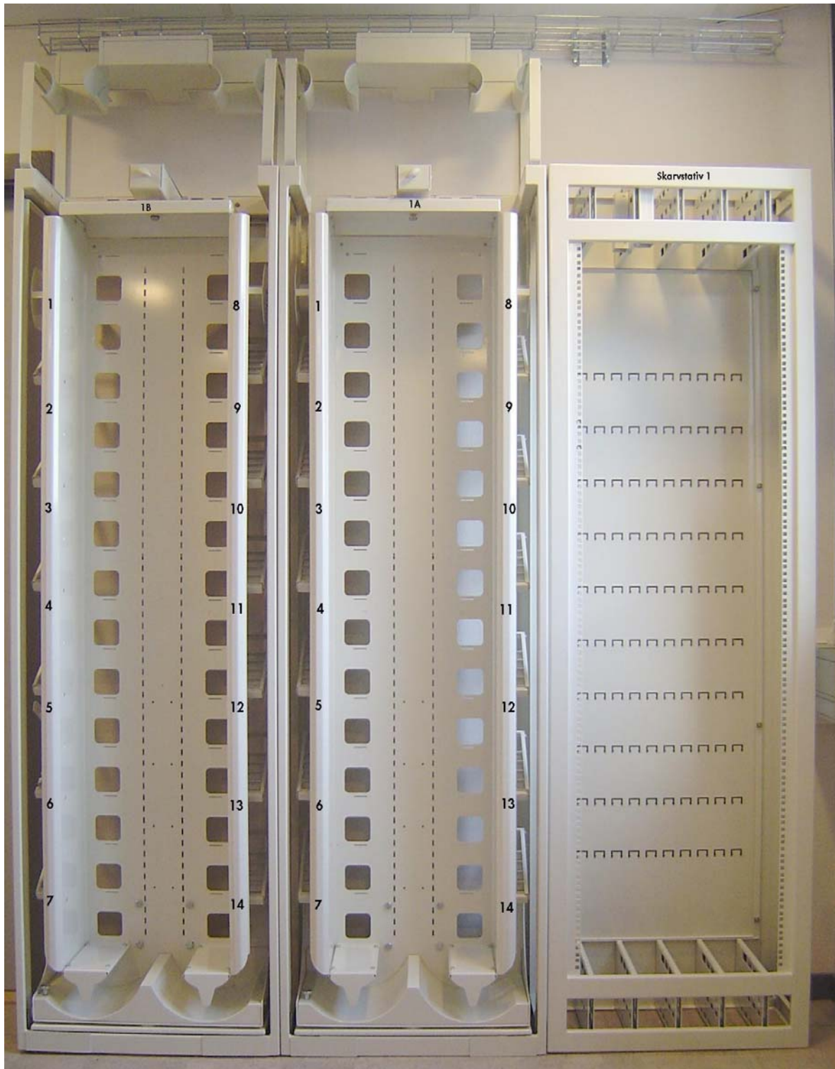
Marking of Patch Frame and Splice Frame
