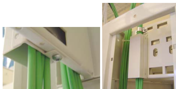
Screwed cable clamp
