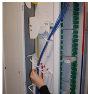
Laying in guides
