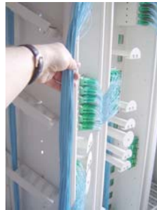
Releasing the patch cord
