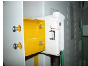
Radius limiter, Locking piece
