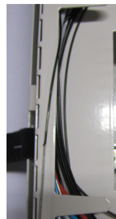
Midspan tub cable 48-fiber together with connection for 48 micro cables ( \varnothing < 2 mm) with micro cable (customer)
