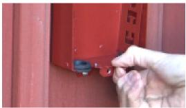
Remove the seal, measure the length of the pipe, and cut it off
