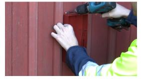
To avoid threading the pipe, there is a seal with a hatch that allows the seal to be removed.
