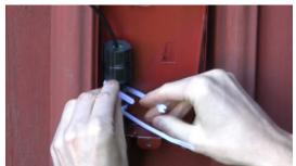
Strip the cable. If it contains yarn, it can be strain relieved on the T-bracket. The yarn can be cut about 6-7 cm, then you can wrap it 3-4 times around the T-bracket. If there is no FRP jacket to clamp onto, wrap the yarn 3-4 times and clamp it with the extra accessory.
