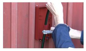
Make a hole in the seal adapted to the size of the pipe/cable and then thread the seal onto it.
